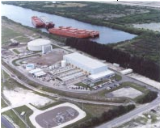
Tampa Bay Desalination Plant Photo courtesy of Aerial Innovations
