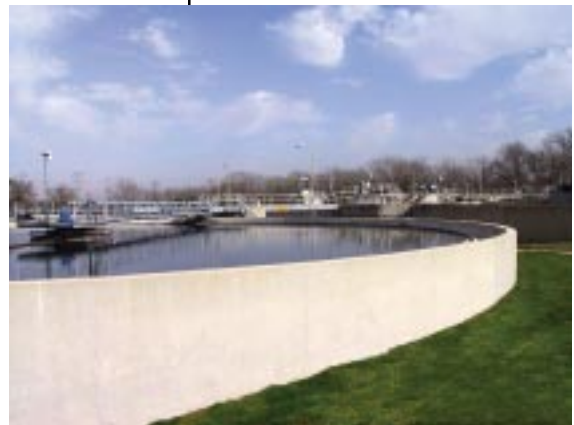
Sugar Land Treatment Plant Photo courtesy of Southwest Water Company
